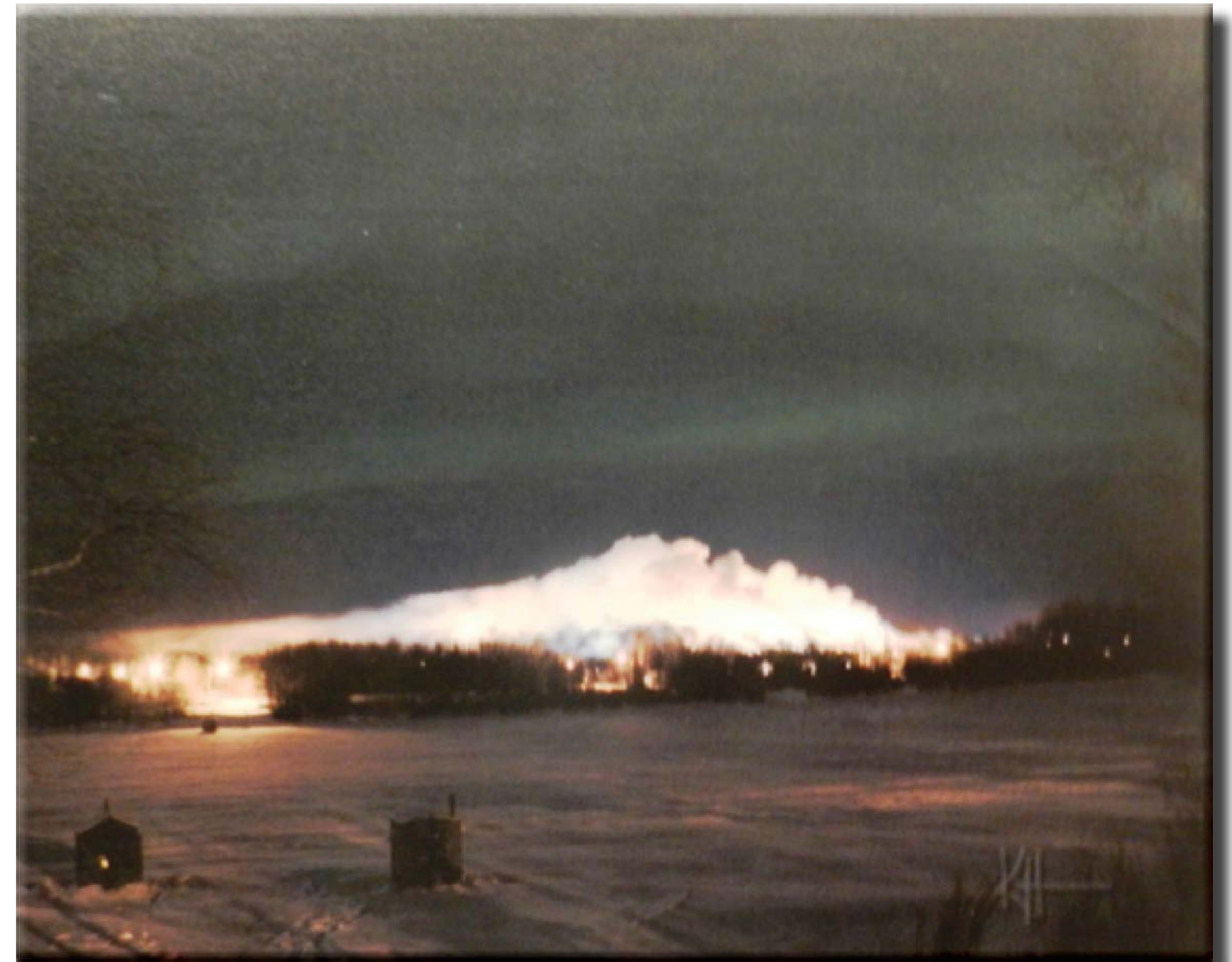
Steam from the Plant
